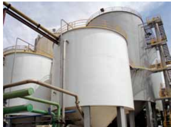
Figure 1. Continuous sugar cane juice fermentation bioreactors
